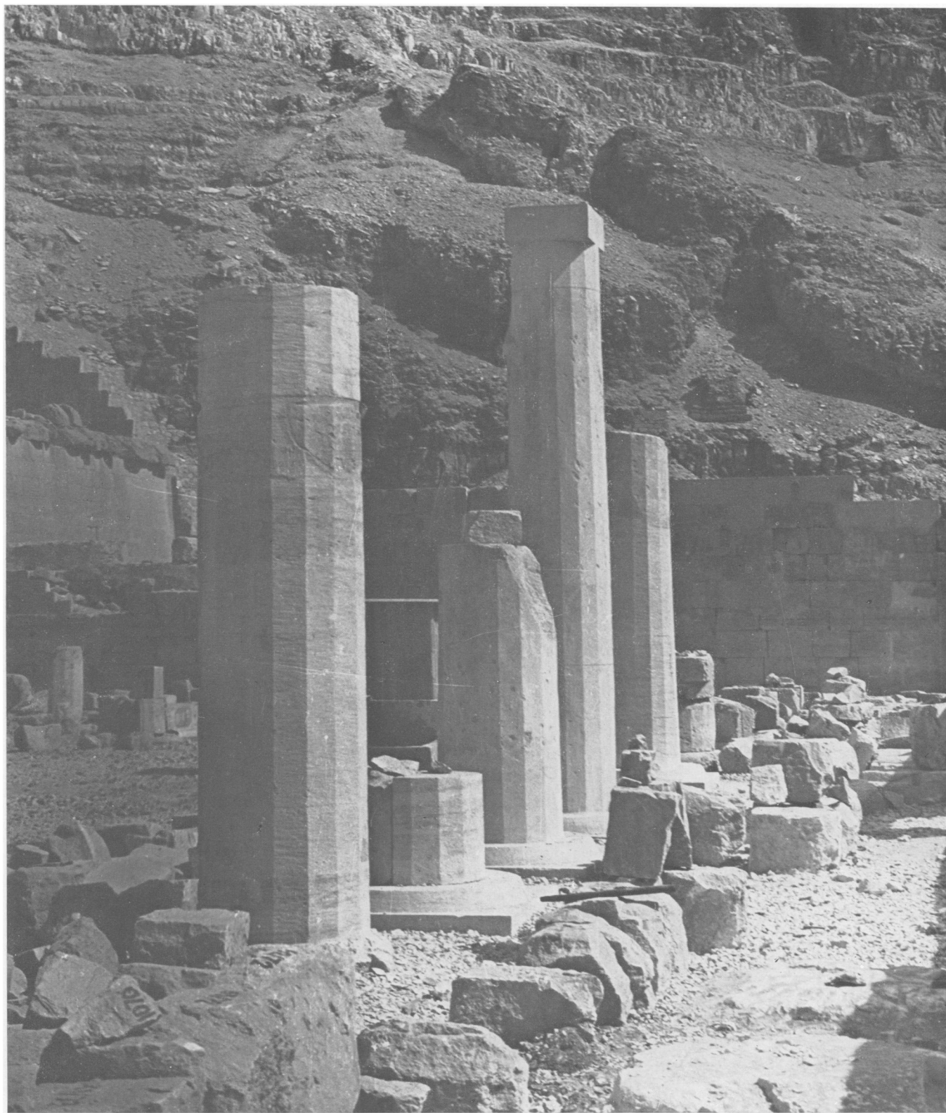
The Queen Hatshepsut Temple. The re-integrated column shafts of the upper courtyard
